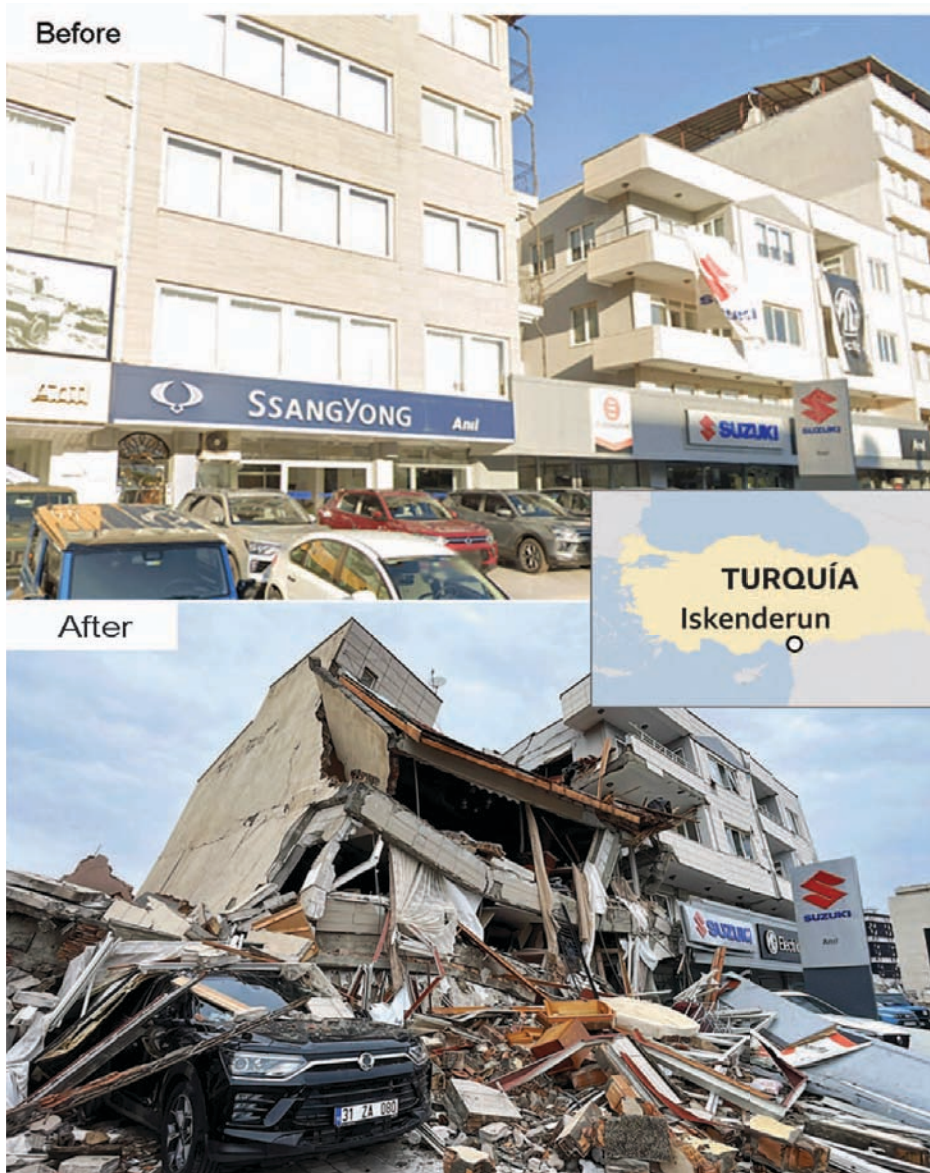
Collapsed building in Iskenderun, Turkey. Source Google, Getty.
